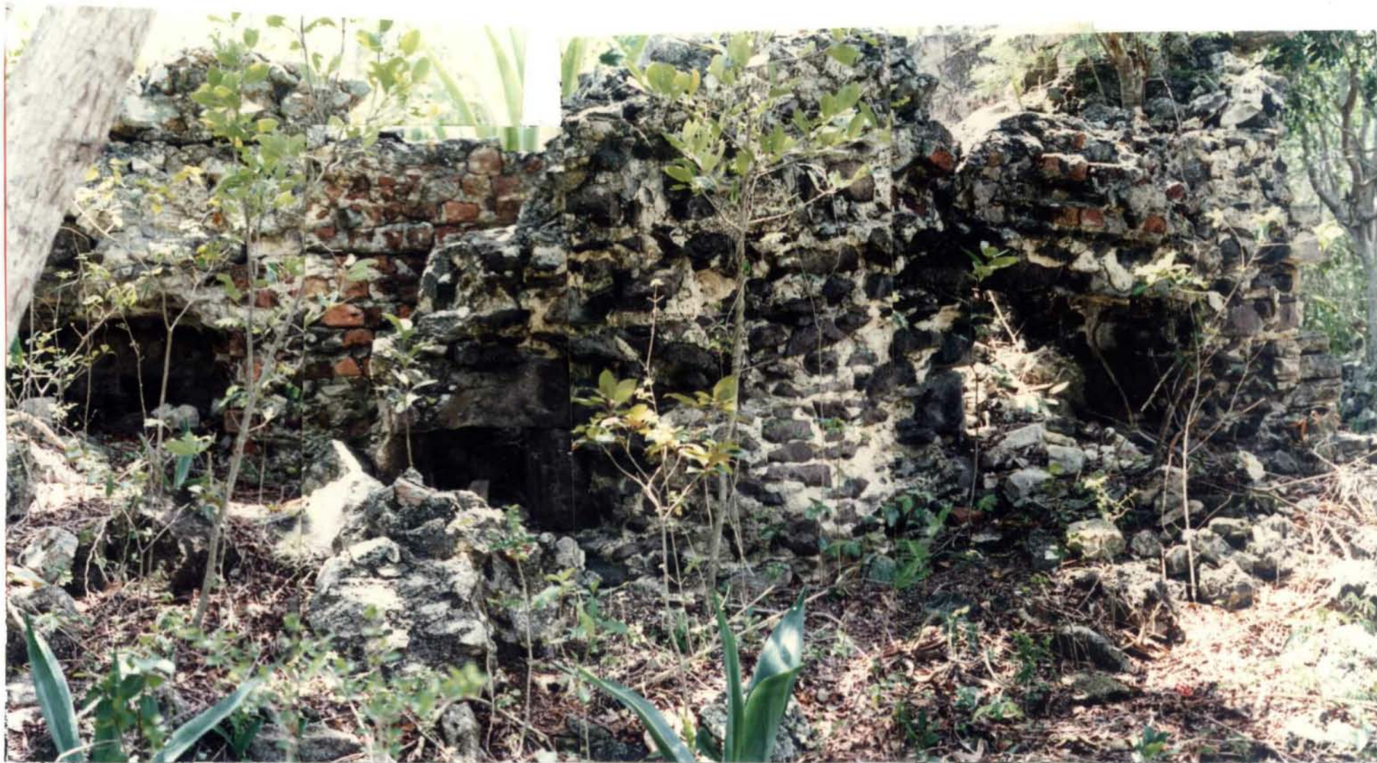
Photo No. 1: Exterior face of north wall with firing gate at left, the vent for draft control in center and the exit of the horizontal flue to the right. Note its finished cover.
