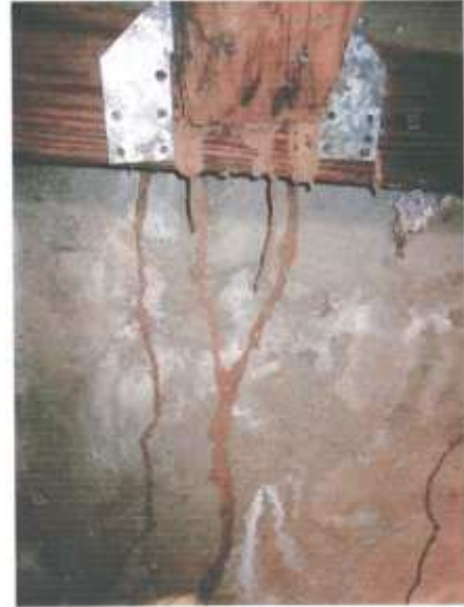
Termite tunnels built on concrete by subterranean termites, connecting the soil to wood
