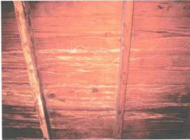
Galleries and damage caused to ceiling of living room, main house, Guana Island by the subterranean termite Heterotermes sp.
